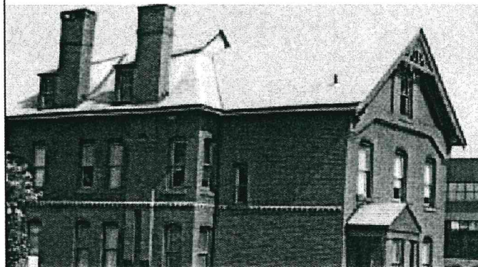
47 Sigourney Street — in danger of demolition
